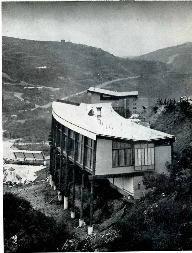
... "nestled" against its hillside lot, the house here displays its slight horizontal curve and stilted Rilco framework ... one entire facade is fenestrated with Fuller glass ... area is Flintridge ...
